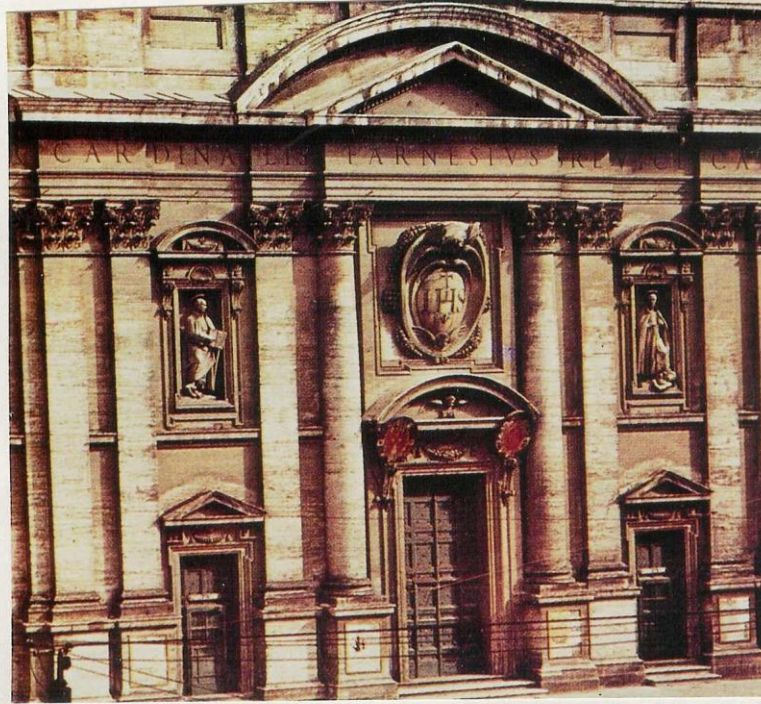
Fig 9. Facade of Chiesa del Gesù in Rome Showing Triangular and Curvilinear Tympana
